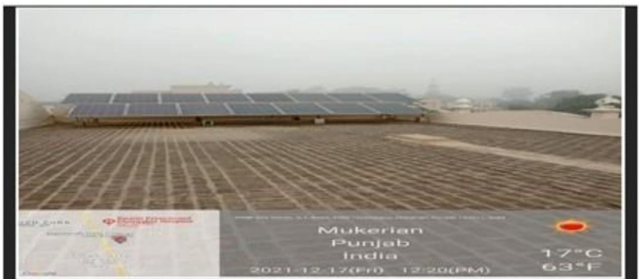
Solar PV on college campus
